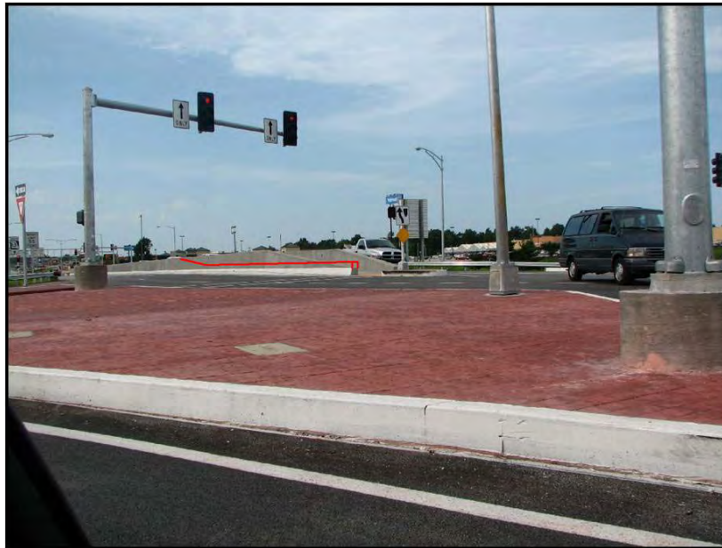
Figure 2.9 The red line shows how the barrier wall could be altered to provide better sight distance
