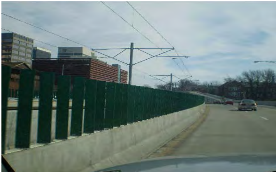
Figure 2.13 Example of a glare screen system
